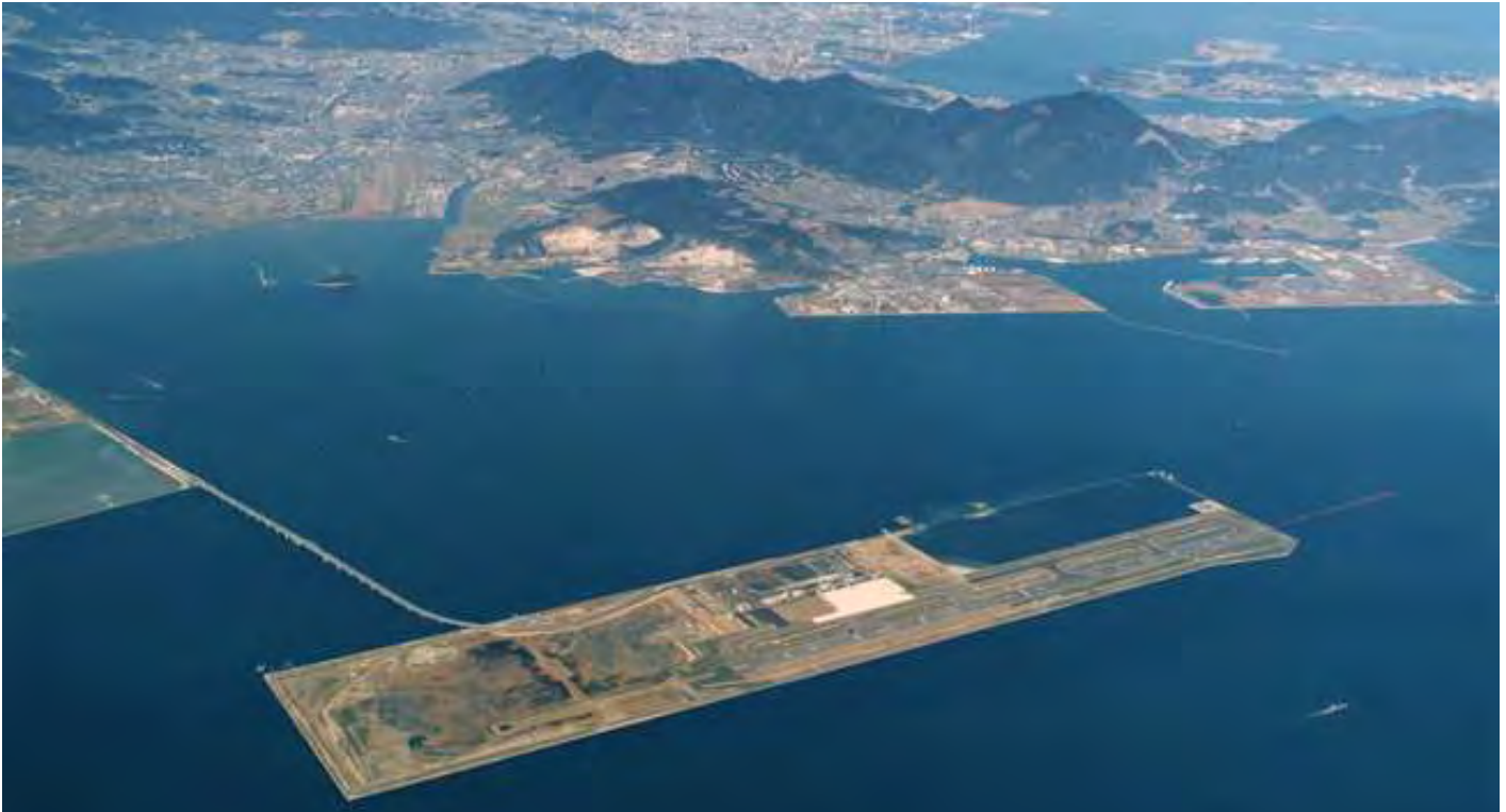
Air view of New-Kitakyusyu Airport
