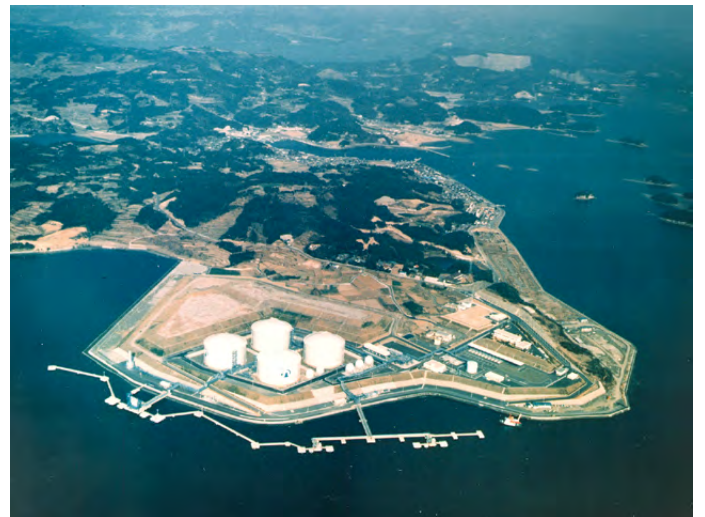
Fukushima LPG base ( KYUSHU L.P.G. FUKUSHIMA TERMINAL Co.,Ltd. ) Fukushima-cho, Matsuura City, Nagasaki
