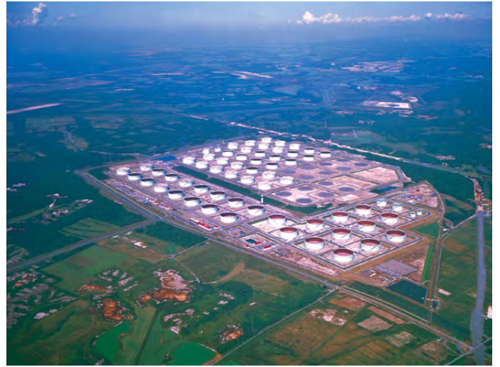
Tomakomai Eastern National Oil Reserve Storage Base Tomakomai city, hokkaido
