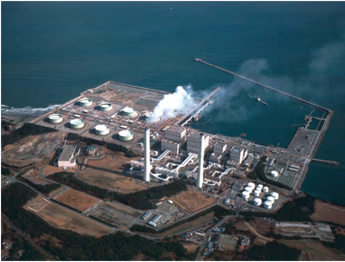
Hirono thermal power plant ( Tokyo Electric Power Company ) Hirono-cho, Futaba District, Fukushima
