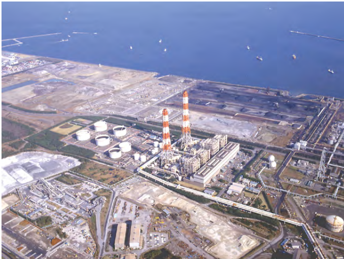
Kajima kyodo thermal plant ( Kashima Kyodo Electric Power Co. ) Kajima City, Ibaraki
