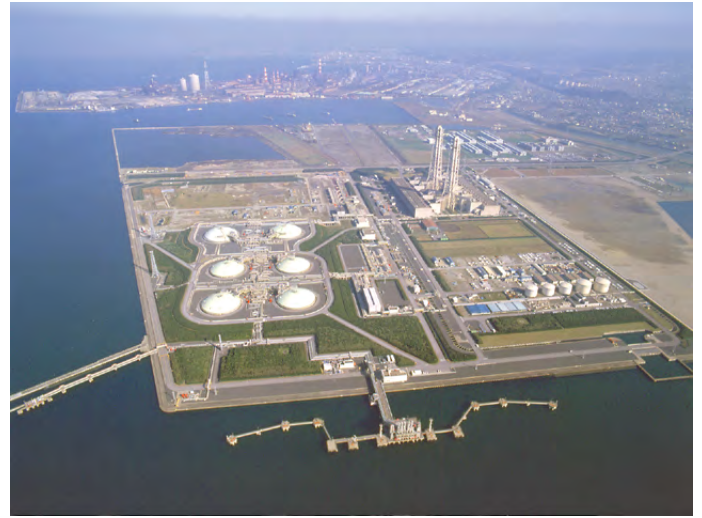
Futtsu thermal power plant ( Tokyo Electric Power Company ) Futtsu City, Chiba
