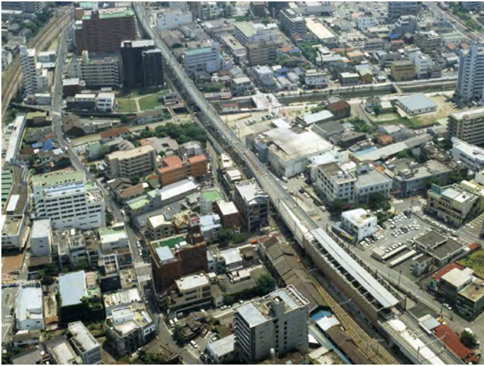
Continuous grade separation for the area around Kashii Station ( Nishitestu Kaizuka Line ) Fukuoka City Completion:2006
