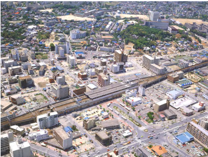
Continuous grade separation for the area around Oohashi Station Fukuoka City Completion:1978
